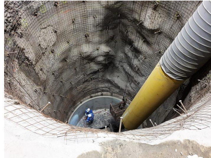
Silo G lining
